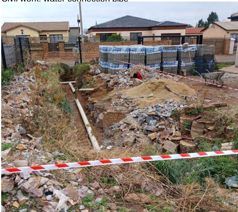
Refuse yard progress: challenges with the rock underground.
