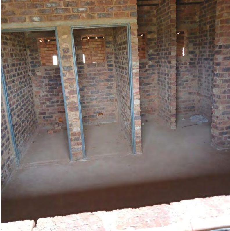
Change rooms: inside view.
