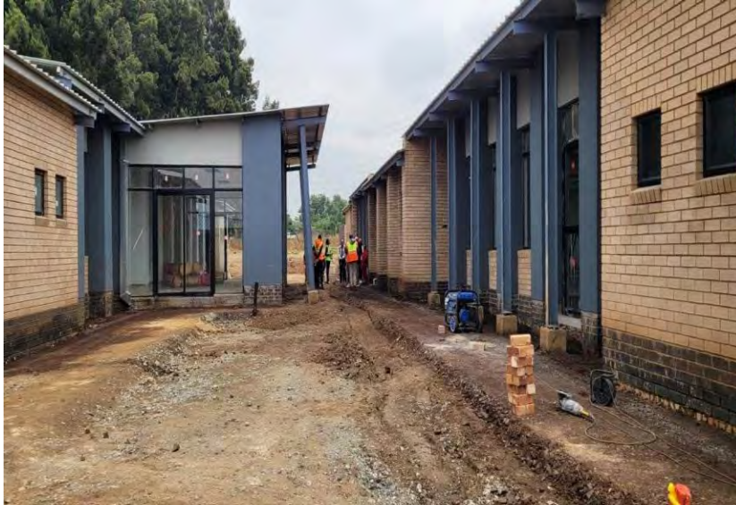
Figure 2: Reiger Park Enterprise Hub and Ramaphosa Vocational Skills Centre Project Office Block B
