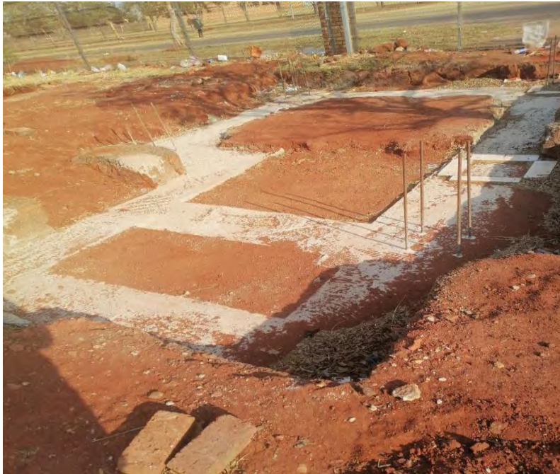
Incomplete guard house: foundation
