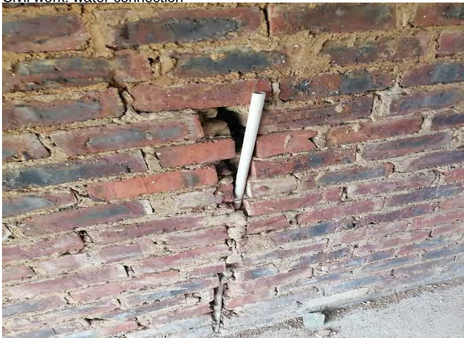
Civil work: electrical work
