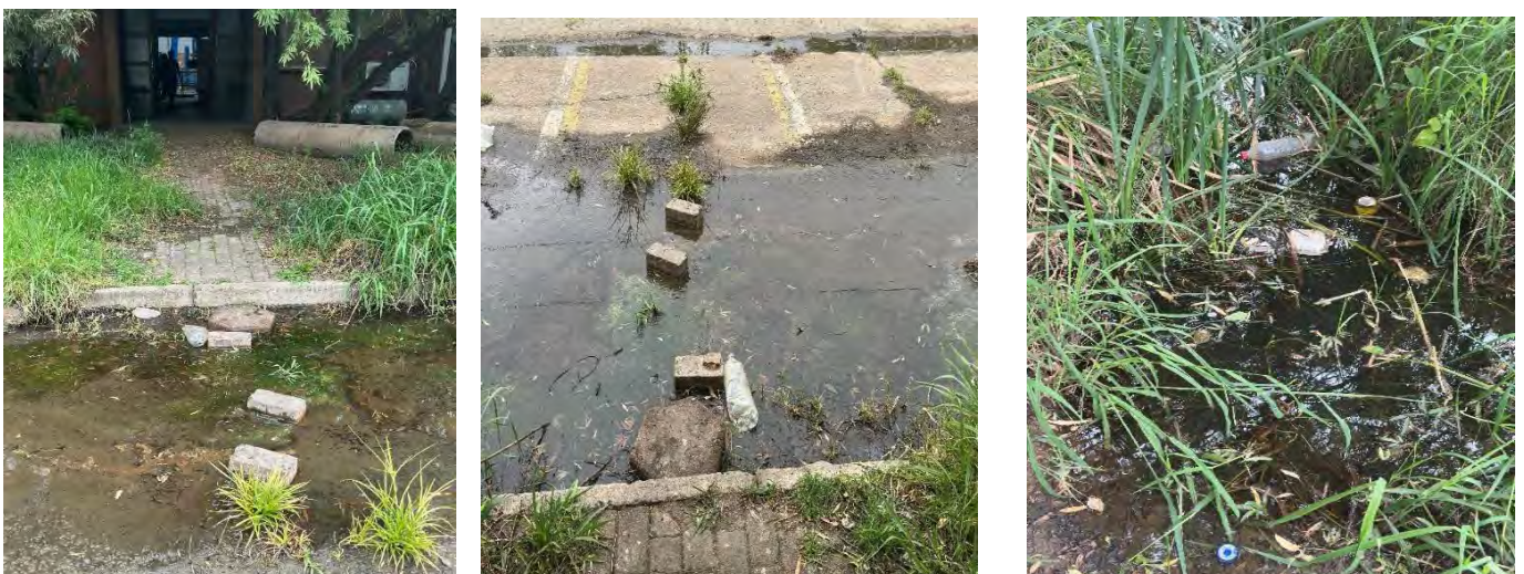
Figure 8: Unmaintained workshop premises
