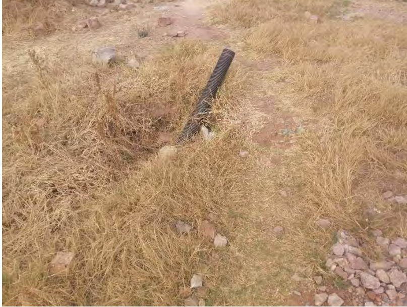
Civil work: water connection pipe
