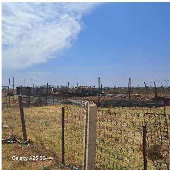
Figure 2: Structure on the farm, erf 6678
